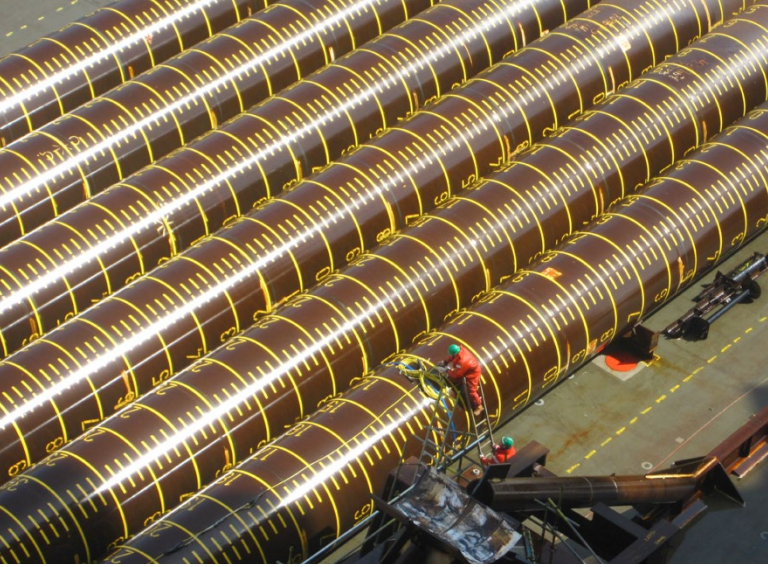
Cable fitting for dynamic pile testing
