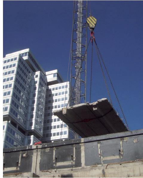
Crane-based demolition at the construction site of the DRV data center.
