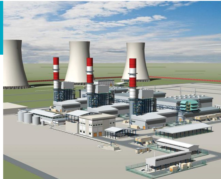
Power plant Siemens in DGEN, India, constructed on over 8,000 foundation piles
