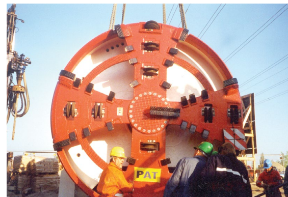
Tunnel boring machine for the waste-water disposal line in Biesdorf-Wassmannsdorf, Berlin
