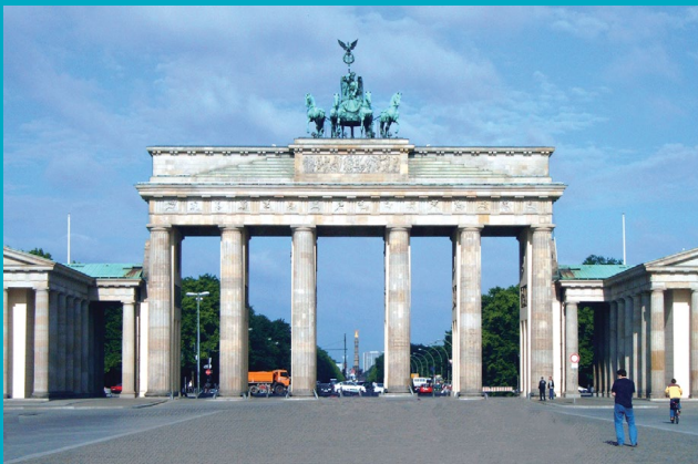
Underpinning the historic foundation of the Brandenburg Gate, Berlin
