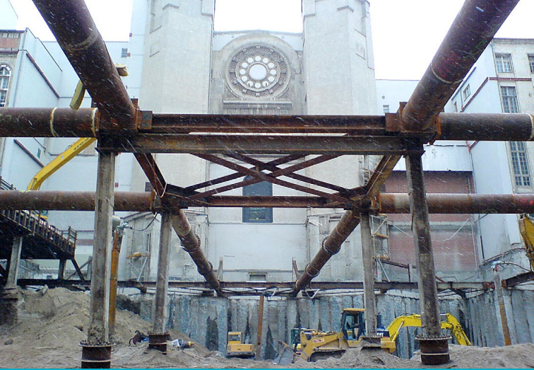
Excavation pit for the National Library in Berlin
