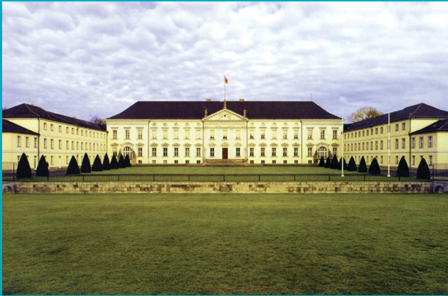
Subsurface construction of a basement by jet grouting at Bellevue Castle, Berlin
