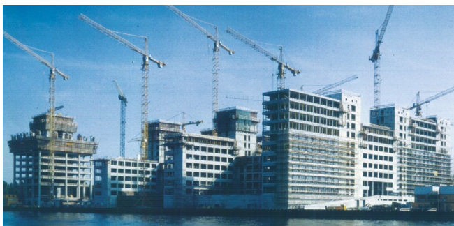
The Treptowers in Berlin, erected on pile – raft foundation
