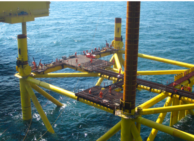
Installation of jacket piles for an Electrical Offshore Substation
