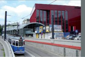
Fast Tram and Opera House Krakow, Poland We have recorded and cataloged the vibrational response of the neighboring buildings for the redesign of vast parts of the underground tram tracks in Krakow. For the directly adjacent newly constructed opera house we have made a prognosis on the structural vibrations and secondary airborne noise in order to design the necessary track insulations along the railroad tracks.
